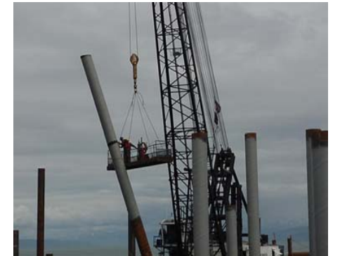
A high-wire act was sometimes necessary as workers cut piles for the new dock. Piles in lengths of 100 to 130 feet were driven in one piece, utilizing a crane that the contractor affectionately called "Thor." Each pile was driven to depth in preparation for placement of pre-cast concrete pile caps and deck panels.
