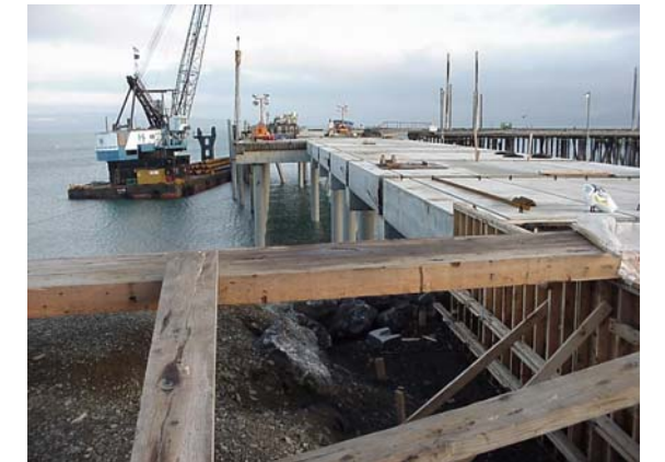
A high-wire act was sometimes necessary as workers cut piles for the new dock. Piles in lengths of 100 to 130 feet were driven in one piece, utilizing a crane that the contractor affectionately called "Thor." Each pile was driven to depth in preparation for placement of pre-cast concrete pile caps and deck panels.
